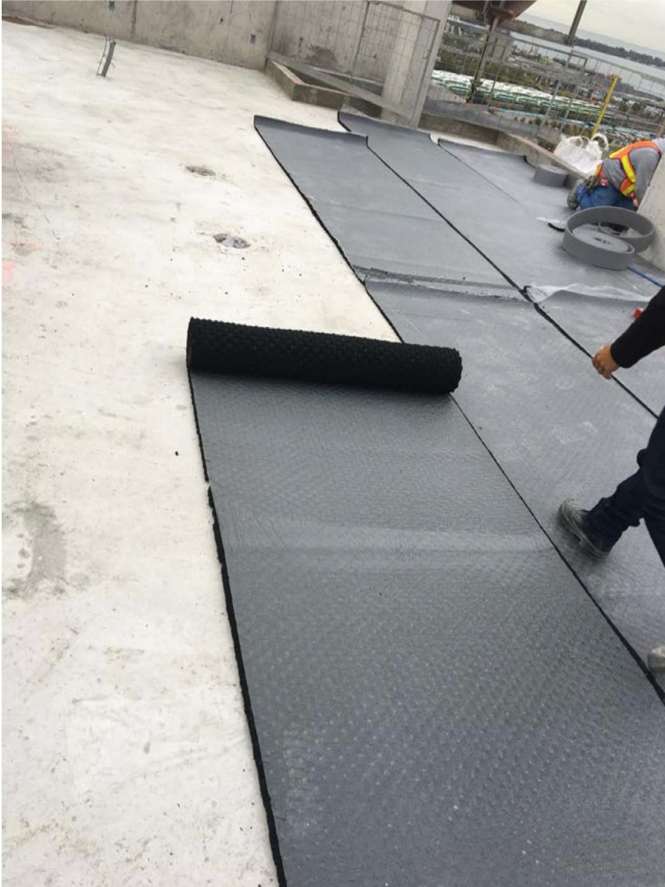
6. Use duct tape or high-quality carpet tape to secure butt joints and seams, and prevent underlayment from moving. If multiple layers of **GenieMat FF** are being used (i.e. **GenieMat FF50**) then only the seams on the top layer need to be taped.
